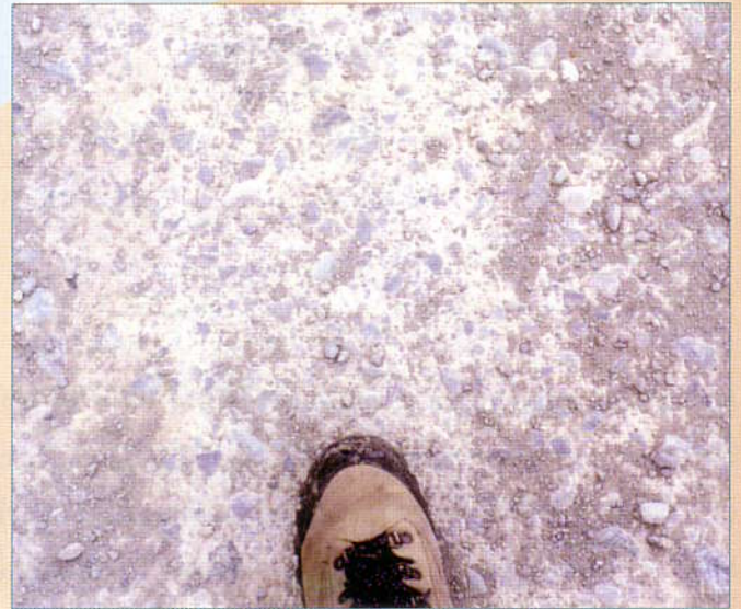
Figure 1 - Well compacted firm road base
