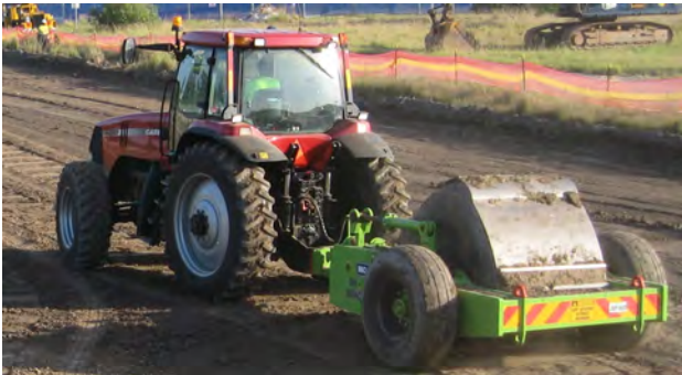
Figure 2. Impact rolling in progress.
